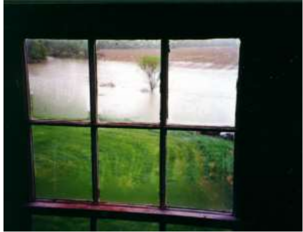
View From Attic Window Showing Extensive Flooding In Old Hoosic Creek Channel Beside Mansion.
